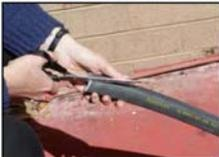
**STEP 2:** Look for 1 metre of pipe insulation (foam rubber) at your local hardware. Domestic water pipes need insulation with a 13mm internal diameter. Cut the insulation foam if it does not have a split already
