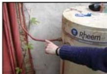
**STEP 1:** Find the hot water pipe at top of hot water system. Heat loss from the tank will be occurring at the outlet.
