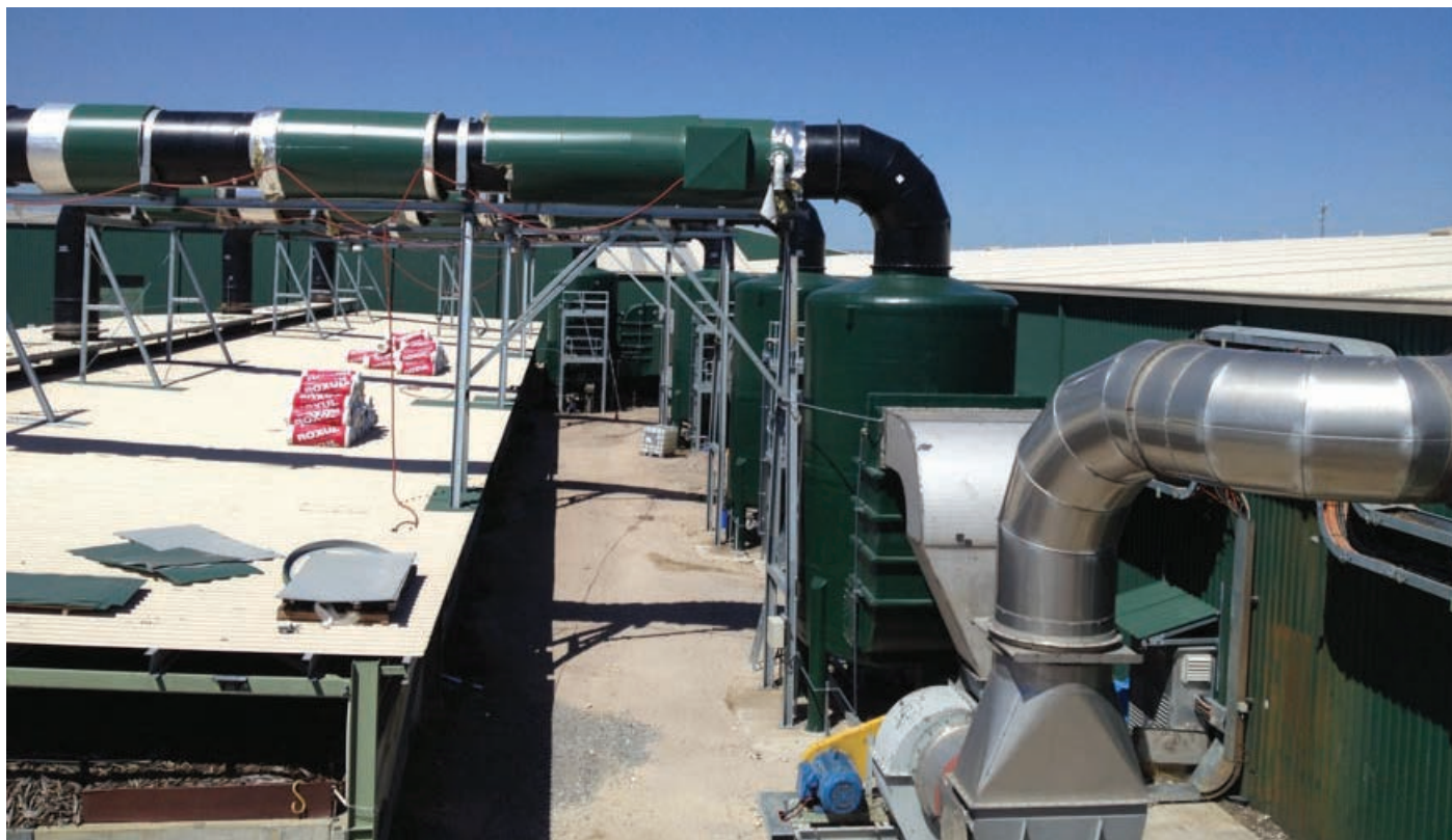
Humidifiers 1-4 complete and acoustic lagging repairs underway.
