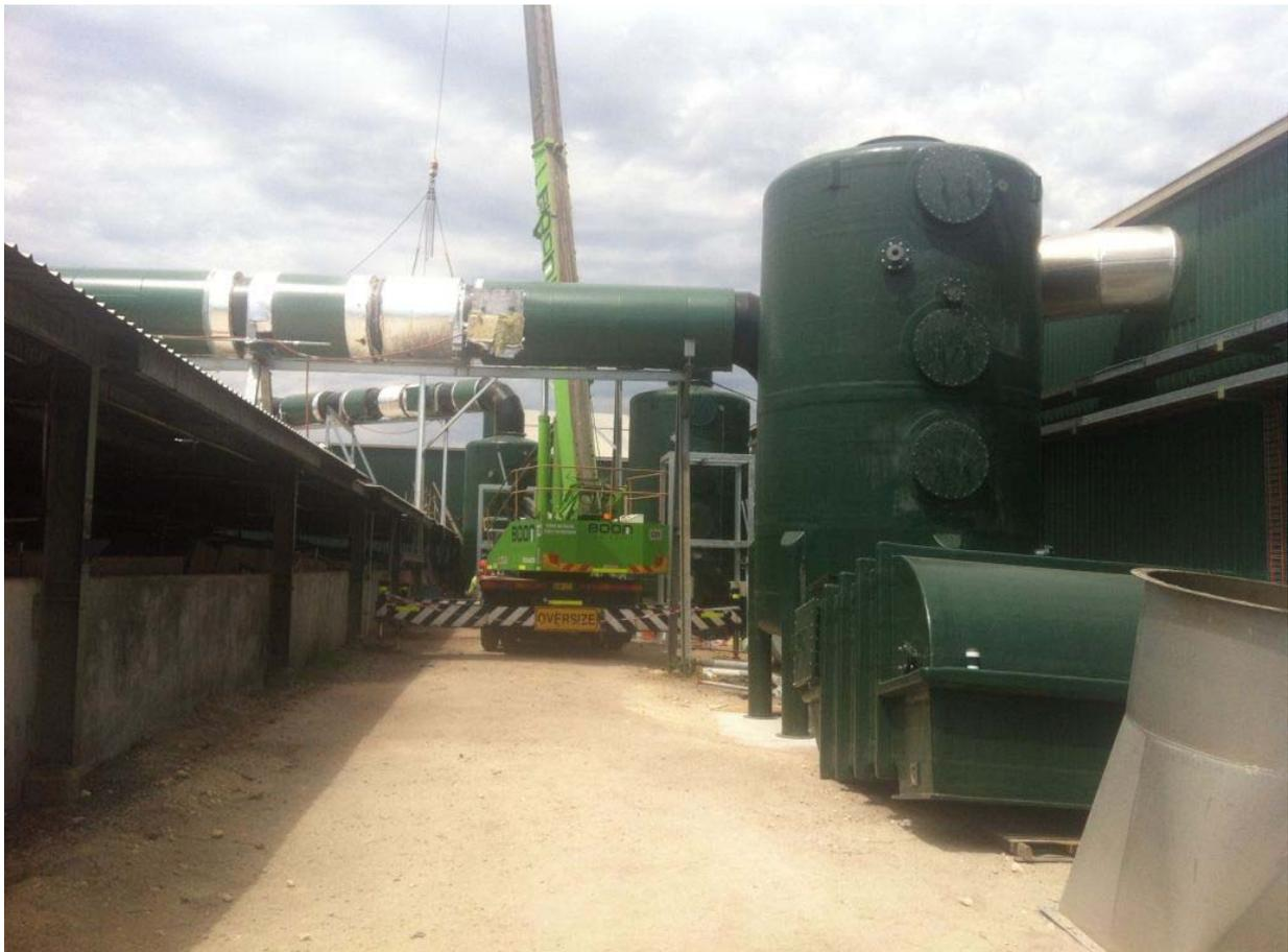
**This photo shows the installation of Humidifiers 4, 3 & 2 on Bio Filter 1.**
