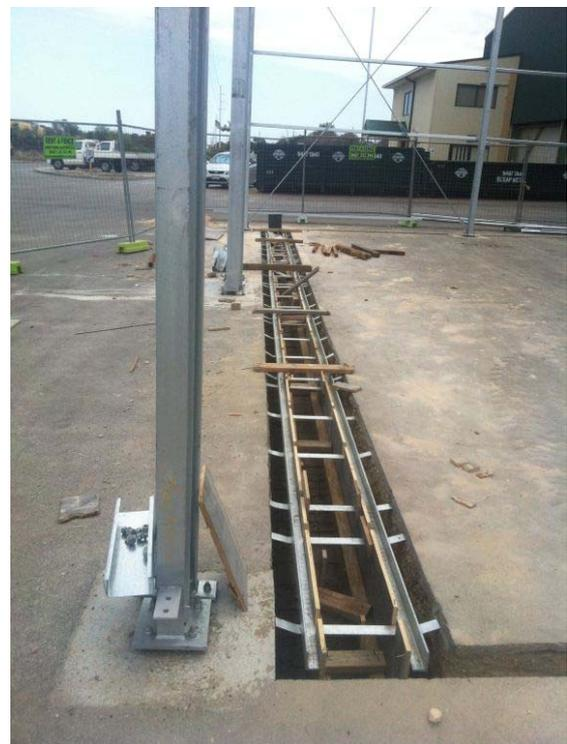
**Footings and framework complete and the floor drain works are underway. Cladding of walls and roof will commence shortly.**
