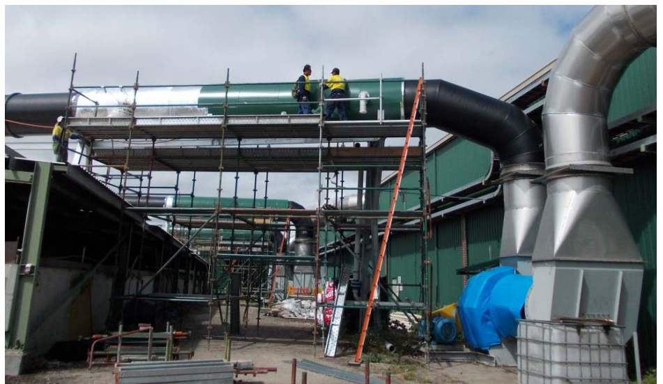
Works well progressed on remaining discharge ducts
