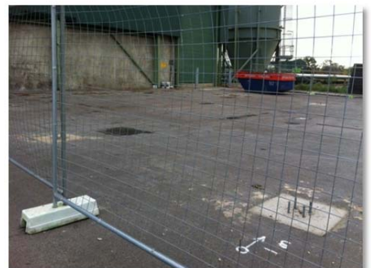
Ground works required for the bin storage shed have commenced
