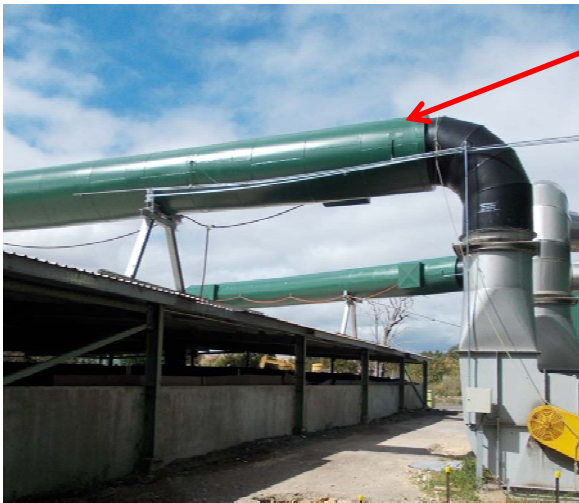
Completed lagging on two of the discharge ducts.
