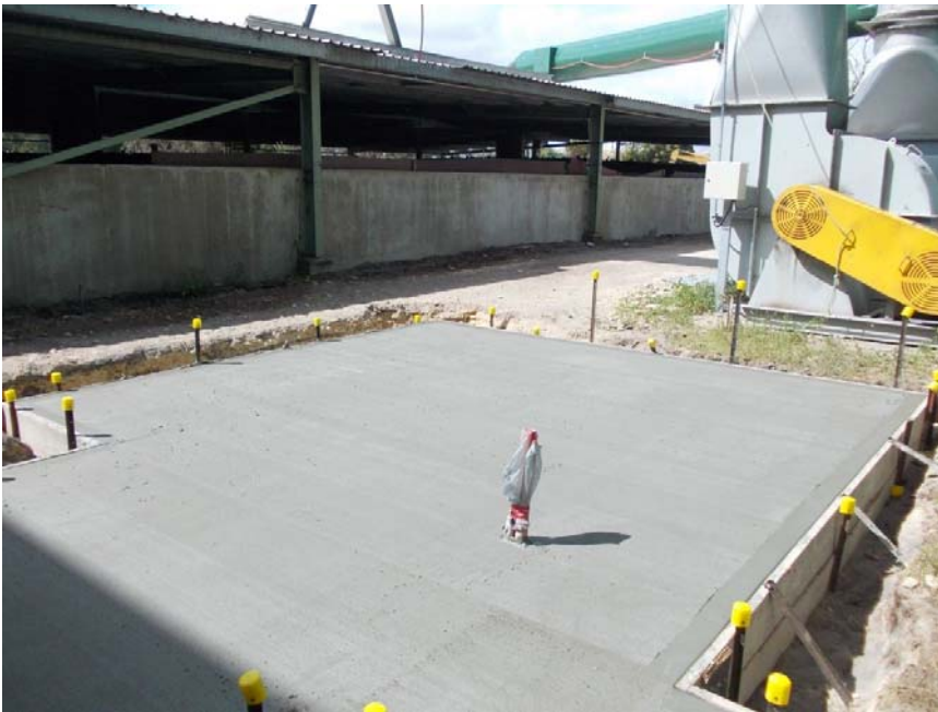
Humidifier foundations have begun
